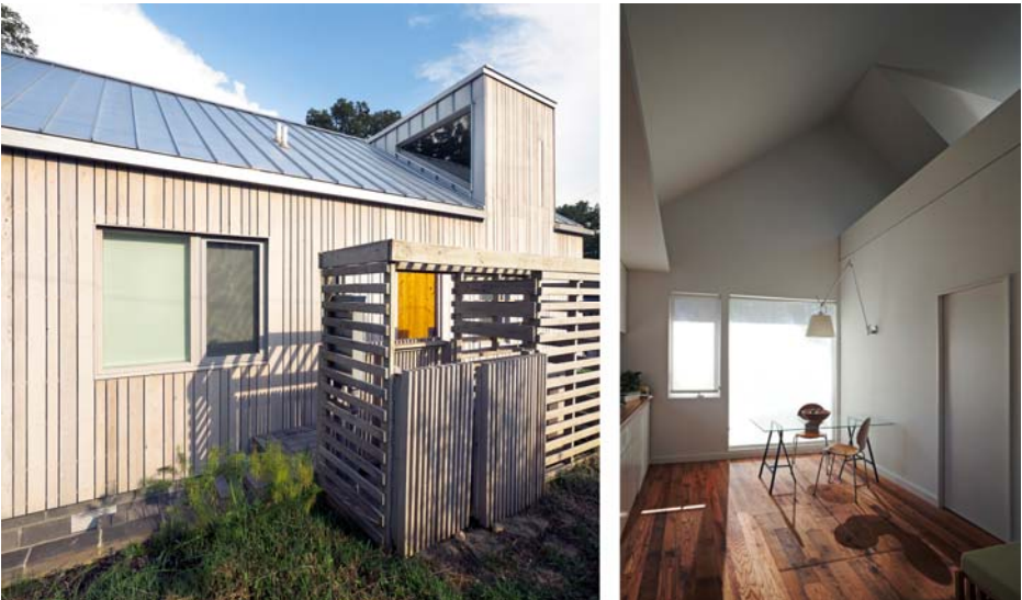
Fig. 8 The dormer on the west side of the home and a view of the interior towards the street. Winter light is allowed to penetrate deep into the space. (photo by Ken McCown).
