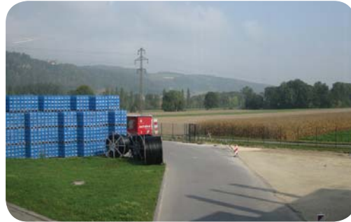
Existing Henniez bottling facility
